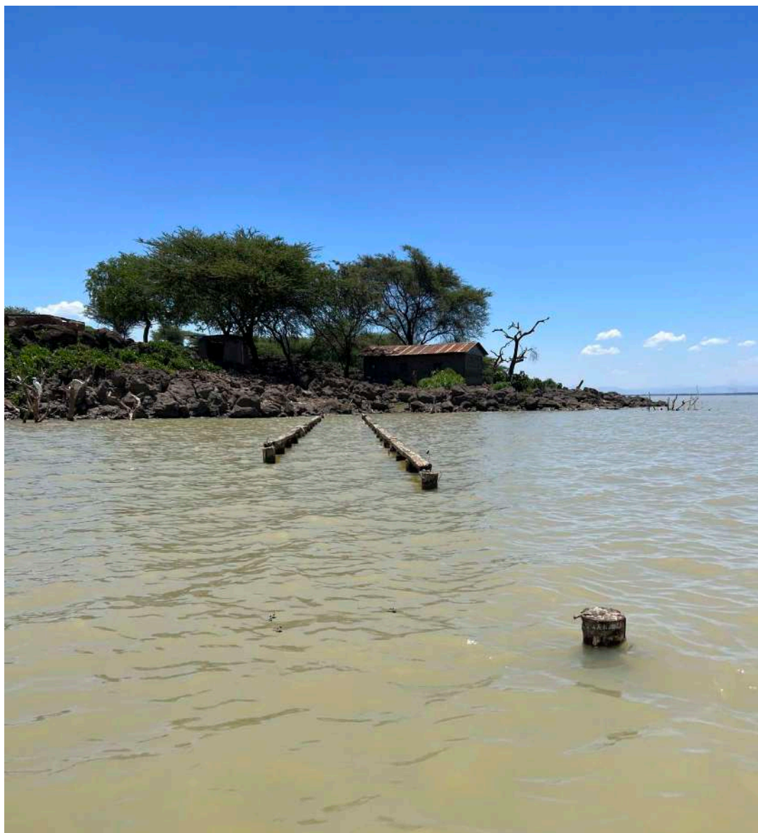
Bridge once connecting two islands now submerged by rising Lake Baringo – Amali Tower/Climate Refugees
