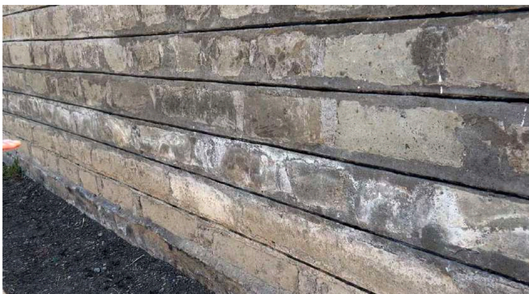
Sebastian Leparyio of BWYO points to the white line on the school wall that marks the flood waterline, Amali Tower/Climate Refugees
